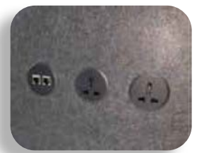
AH Meyer Power & RJ45 Data Point
